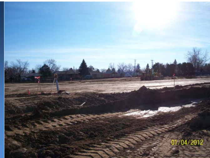
Stockpiled impacted soil and remnants of remediation system from old gas station, ready to be disposed of offsite.
