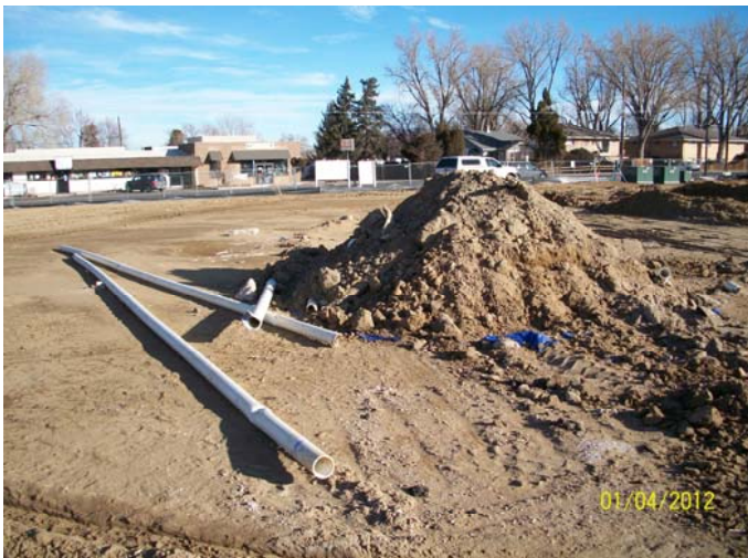
Stockpiled impacted soil and remnants of remediation system from old gas station, ready to be disposed of offsite.
