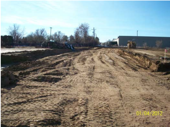
Vance Street road grading.
