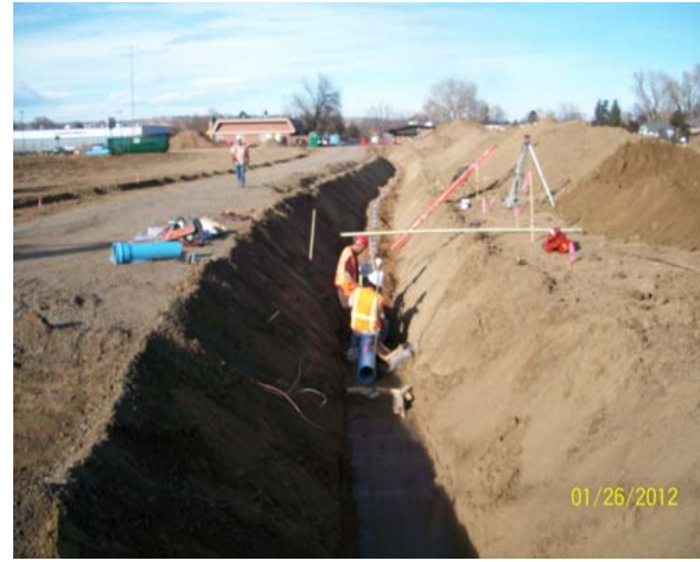
Vance Street water line installation, ready for backfill.
