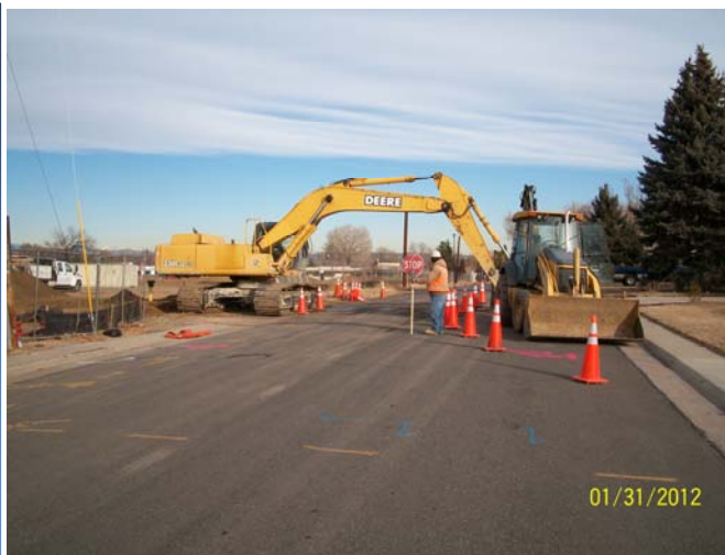
Exploratory excavation for water line tie-in on Upham Street.
