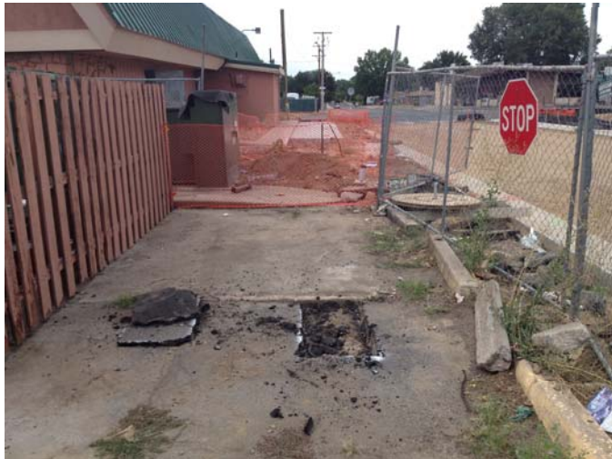
Panda King restaurant trash enclosure relocated for new sidewalk.
