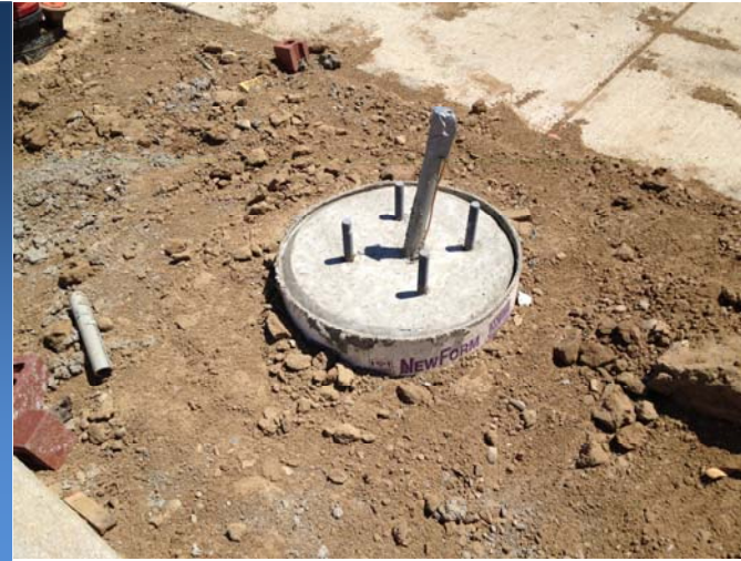
Concrete bases for street and pedestrian lighting installed.
