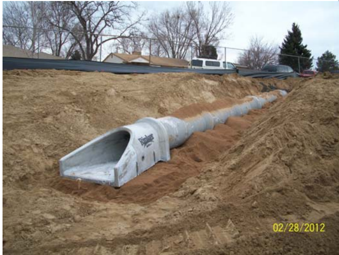
Storm water line and outlet structure from Wazee property into the storm water pond. Awaiting backfill.
