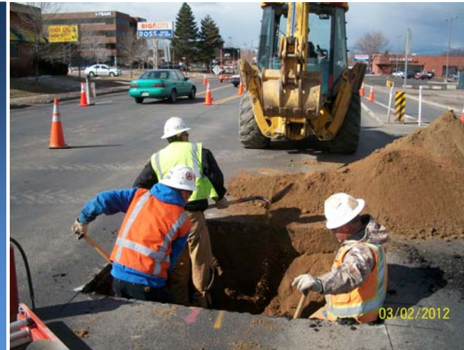
Workers tying gas lines in to gas main on 44 th Avenue.
