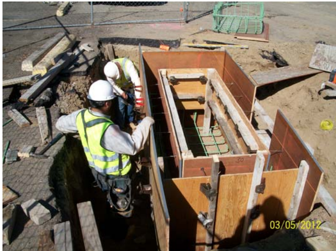
Workers forming storm water inlets on Vance street.
