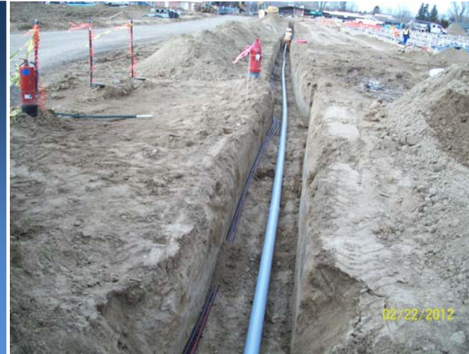
Storm water line and outlet structure from Wazee property into the storm water pond. Awaiting backfill.
