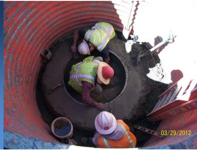
Storm Sewer tie-in to main on Vance street. Setting concrete forms for manhole.
