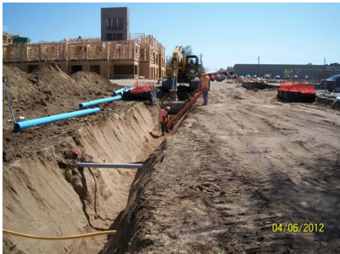
Trench for water line completion on Vance street.
