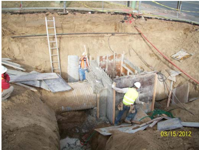
Storm Sewer tie-in to main on Vance street. Setting concrete forms for manhole.
