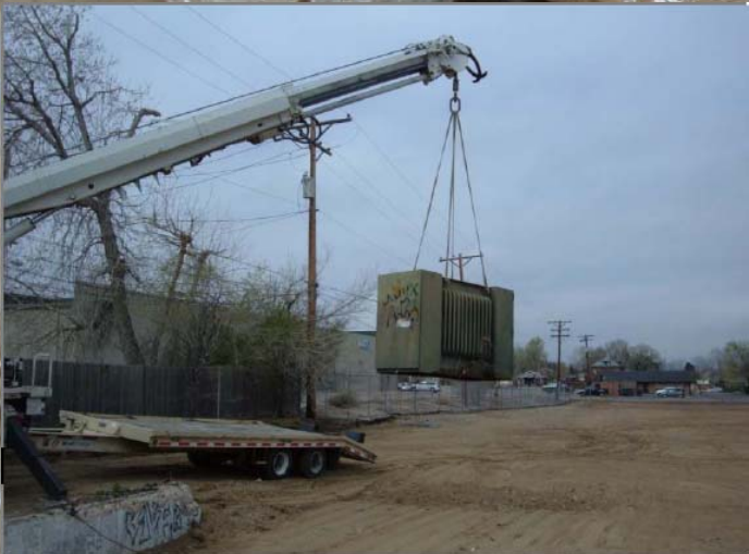
Xcel Energy removing ground transformer from site.
