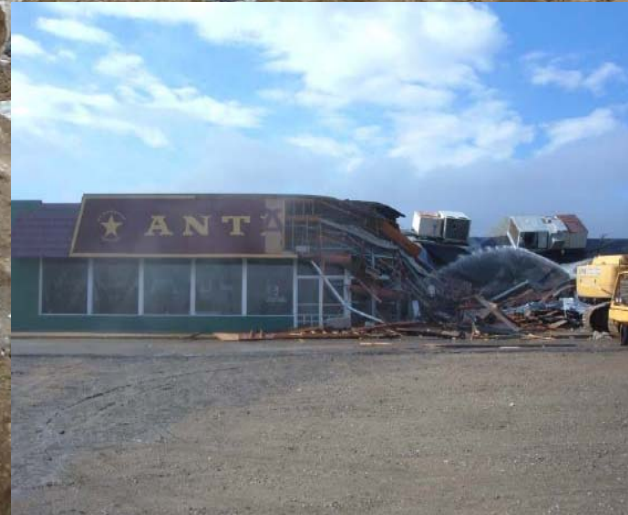
Demolition activities at former antique mall.
